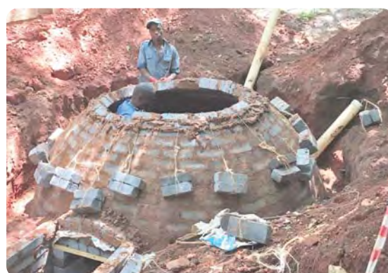
Construction of a GenderCCSA biogas plant in Eastern Cape. Photo: GenderCCSA
