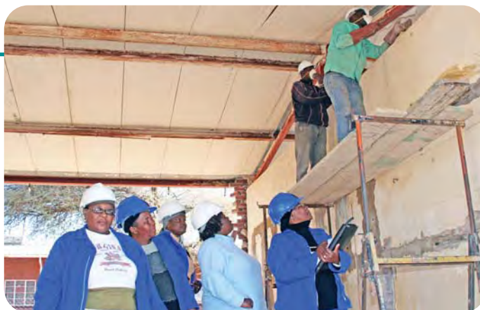
Women working at a construction site in South Africa.
