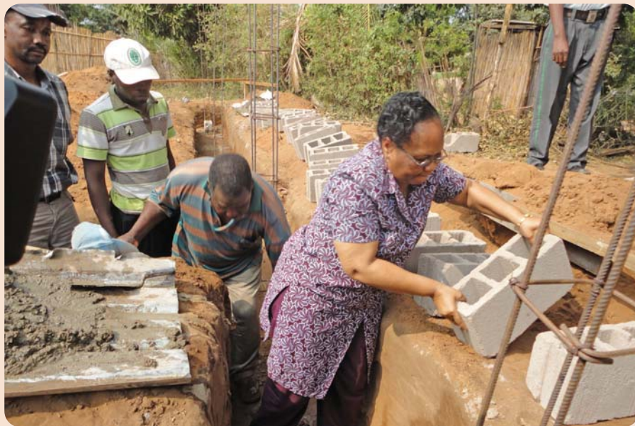
Rita Bento Muianga, Chairperson of the Xai-Xai City Municipal Council, laying bricks Photo provided by Xai-Xai Municipal Council
