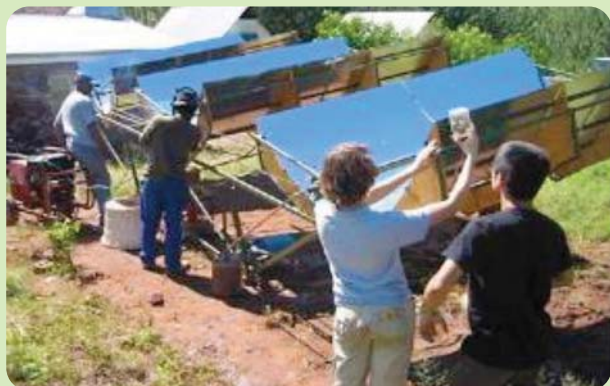
Students help install solar panels as part of a 2014 solar project in Lesotho. Photo: Courtesy of MIT News
